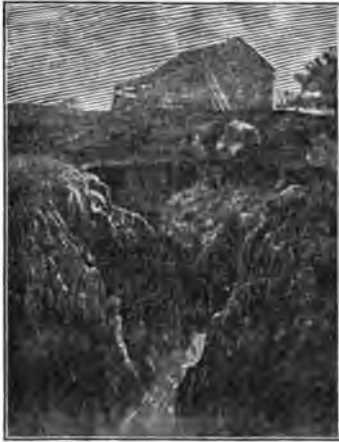
FIG. 40.—Erosion in Mississippi Table Lands, causing destruction of agricultural value both of Uplands and Valleys. (McGee, 12th Ann. Rept. U. S., 1890-91.)
